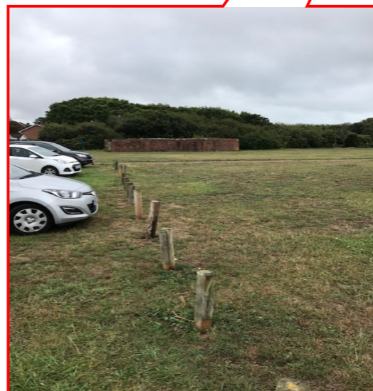
Dragon's teeth need updating some can be picked out by hand
